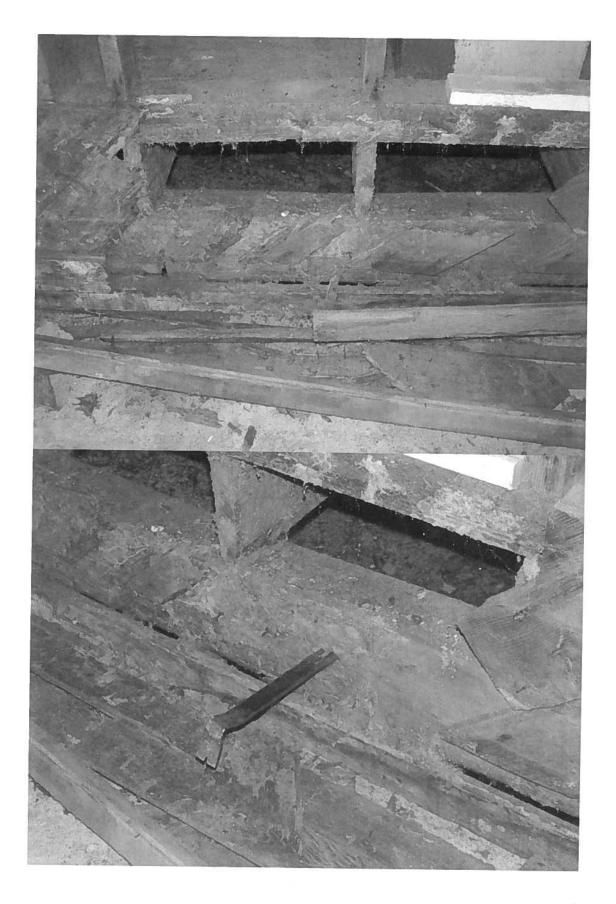
The construction bar in the previous picture was pushed by hand into the 6" x 10" girder. The damage to the wood in these pictures was done by a combination of insect activity and fungal infestation. There is so much damage to the west wall that the wall is in imminent danger of collapse.
